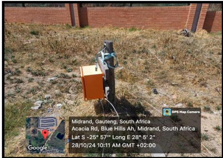
Figure 17: The Installed Boreholes
