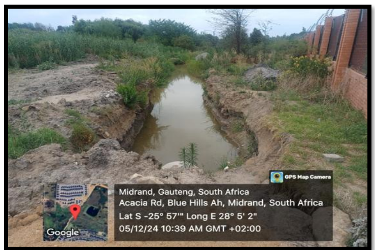
Figure 10: The Installed Culvert
