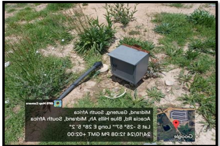
Figure 18: The Installed Boreholes
