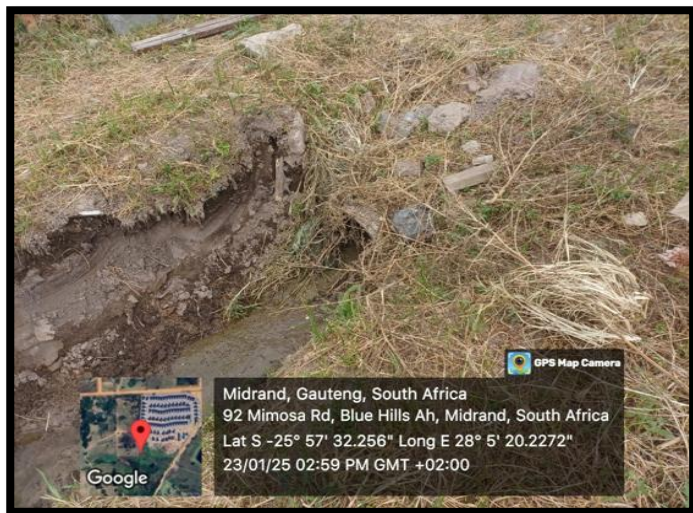
Figure 7: The Culvert installed within the buffer of the Wetland
