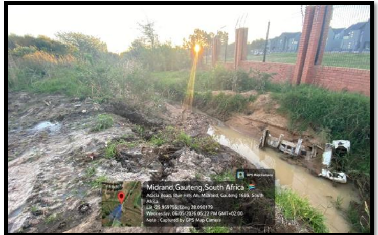
Figure 6: The section where the Culvert is installed
