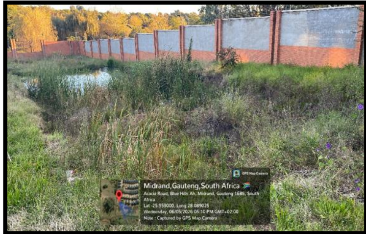
Figure 5: The Back Section of the Boundary Wall
