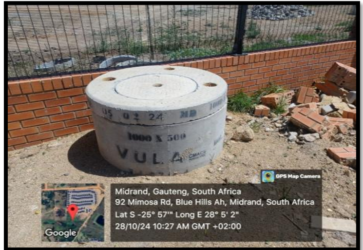
Figure 14: The Installed Manhole
