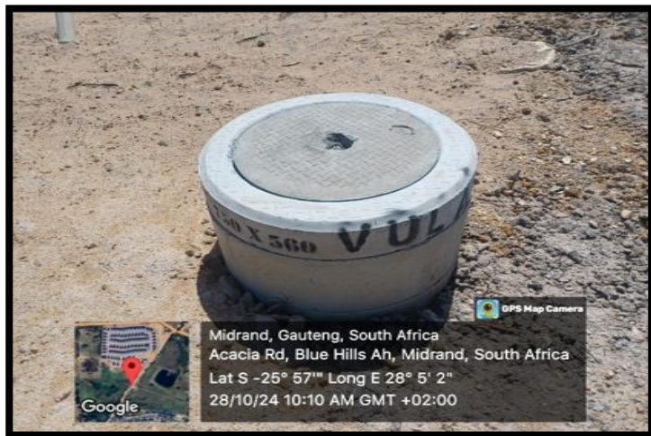
Figure 15: The Installed Manhole
